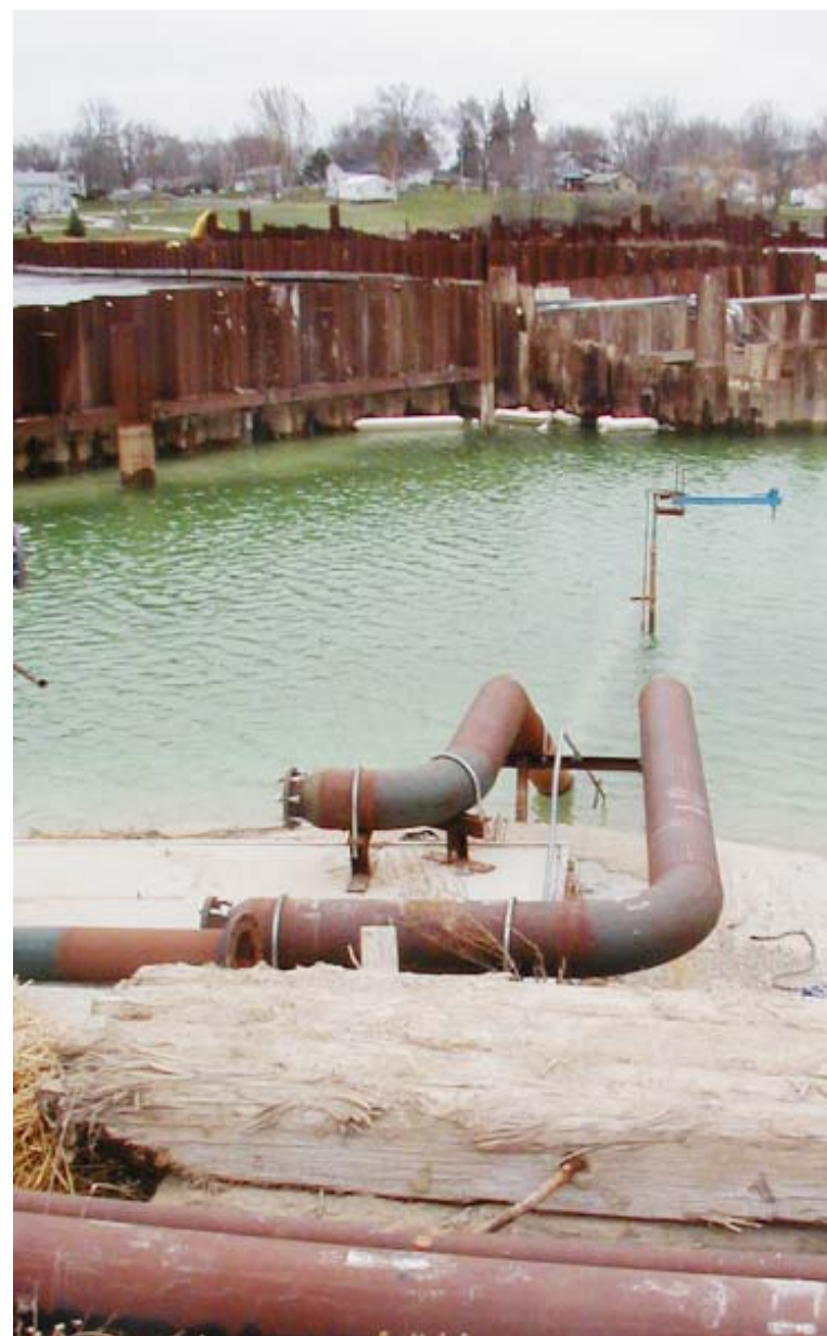
Dewatering Cells in the Pine River (2003)
