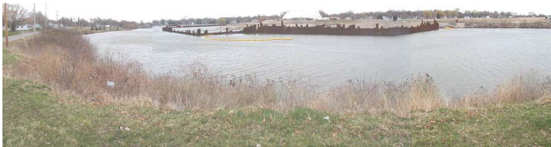
View across the Pine River to the Velsicol Chemical Corporation Superfund Site (2003)
