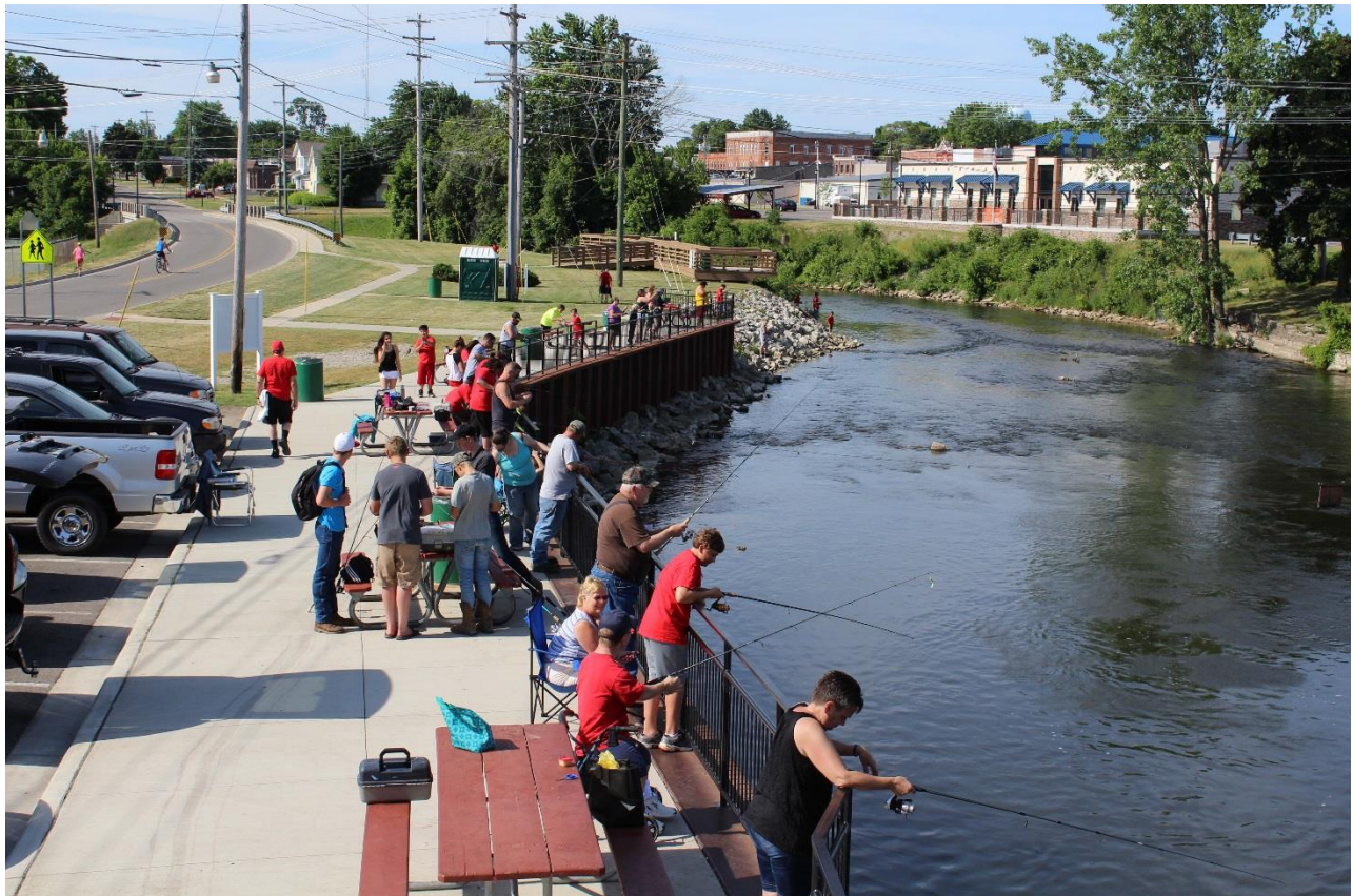
A view of Barnum Park during the Fishing Derby, along the bank of the Pine River, showing bank stabilization project.
