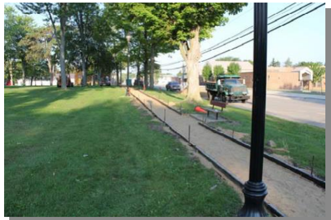
Installation of new sidewalks in Clapp Park.
