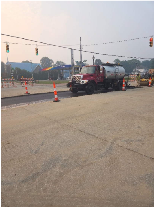
Photo 1: MDOT LAP – M-46/Main Street Sanitary Sewer and pavement repair completed.
