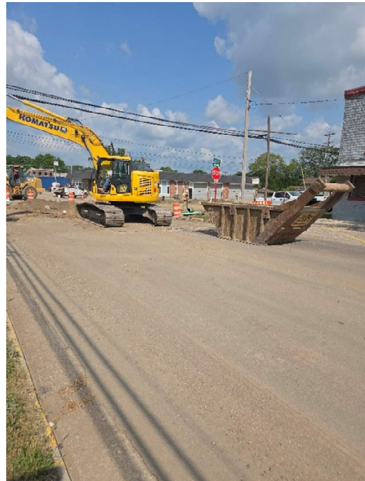
Photo 2: MDOT LAP – Storm sewer placed at Saginaw/Main Street
