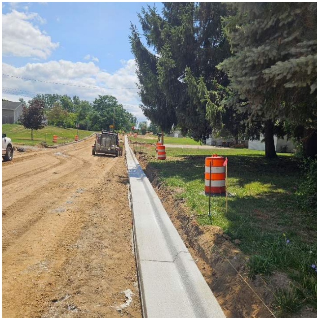
Photo 3: Phase #1 – Concrete Curb and Gutter placed on S. Mill Street.
