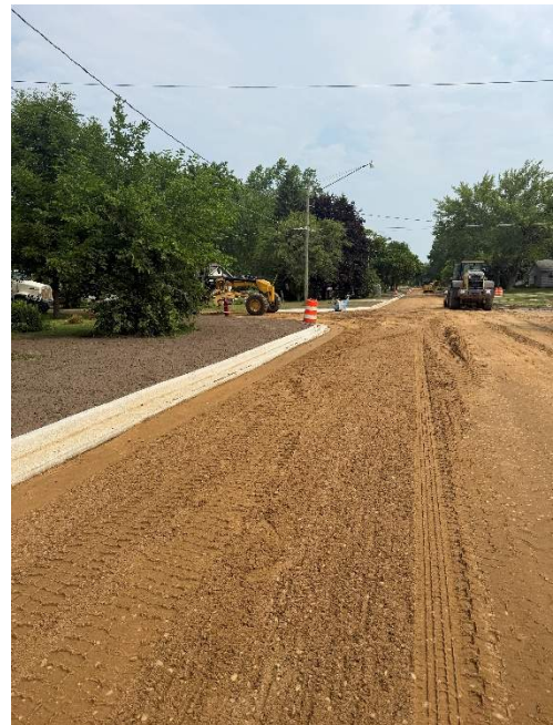
Photo 4: Phase #1 – Topsoil placed on S. Mill Street and road grading started.
