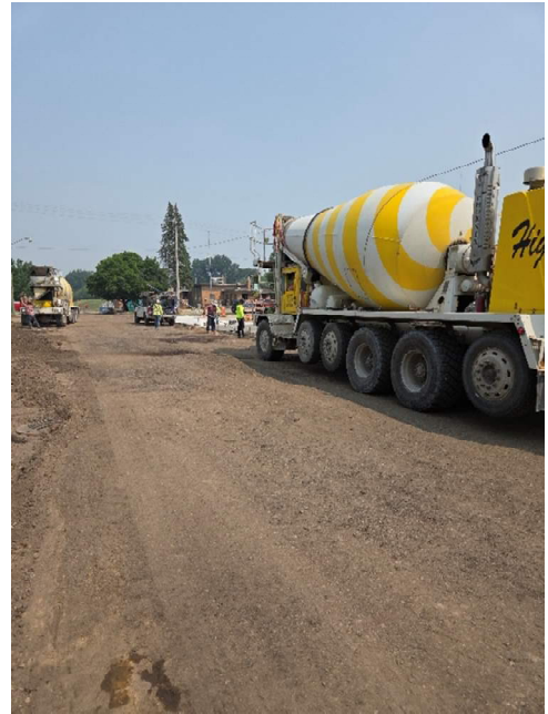
Photo 2: Phase #2 – Concrete driveways, sidewalk, and curb placed on E. Prospect.
