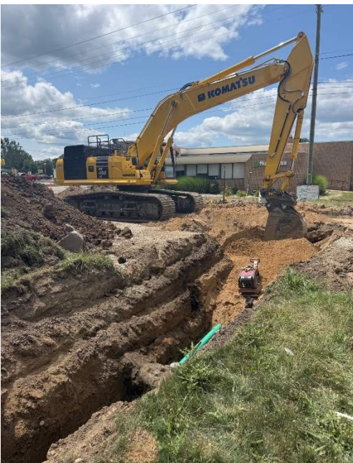
Photo 3: MDOT LAP – Sanitary Laterals installed on N. Main Street
