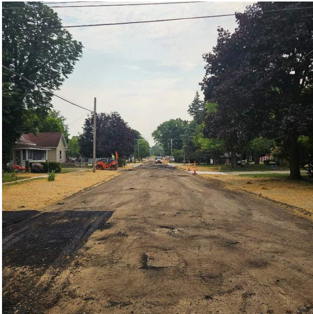
Photo 3: Phase #2 – Restoration completed on E. Prospect and Corinth Street.
