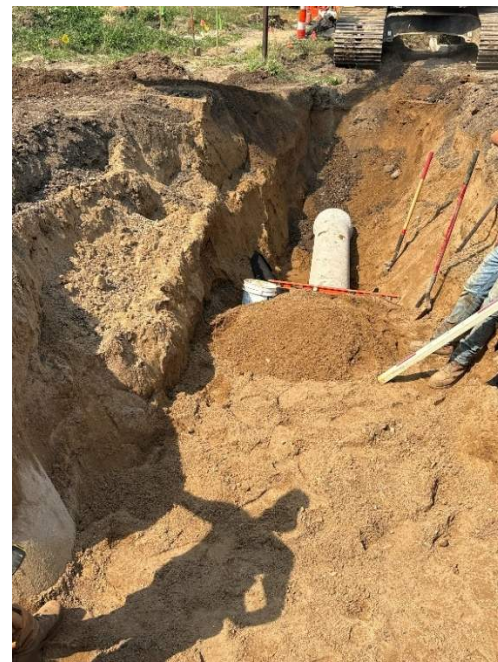
Photo 4: MDOT LAP Storm sewer placed at Center/N. Main Street.
