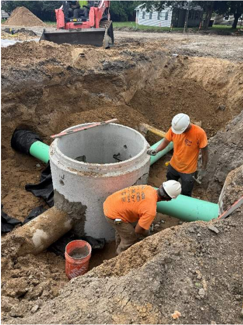
Photo 1: Phase #2 – Storm sewer placed at E. Prospect & N. Clinton
