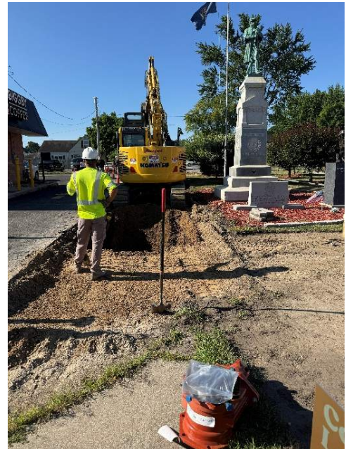
Photo 4: Phase #2 – Water Main Installation started on S. Mill Street beginning at M-46.
