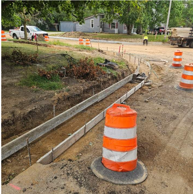
Photo 1: Phase #1 – Storm Sewer catch basins adjusted for curb and gutter.
