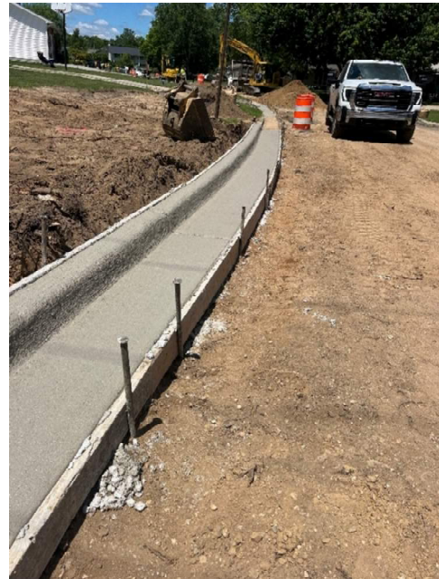
Photo 4: Phase #1 – Concrete Curb and Gutter and driveways placed on Essex.
