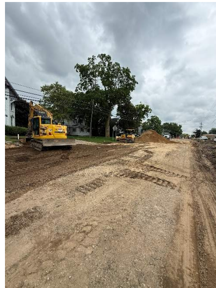
Photo 4: MDOT LAP Sanitary laterals installed on N. Main Street.
