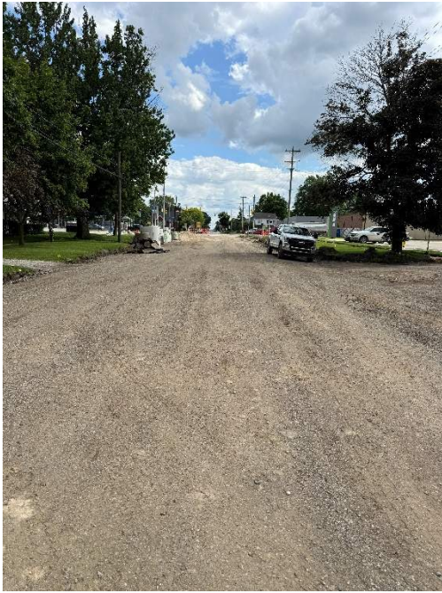
Photo 1: MDOT LAP – Road pulverized and removals completed.
