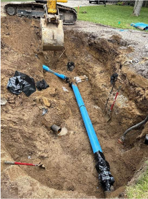
Photo 1: Phase #2 – Water Main tie-ins finalized on E. Prospect St.
