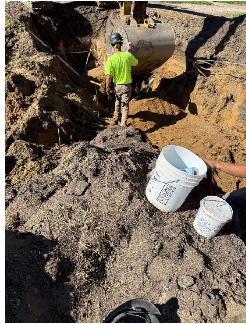
Photo 2: Phase #2 – Water main and services placed on Corinth Street.
