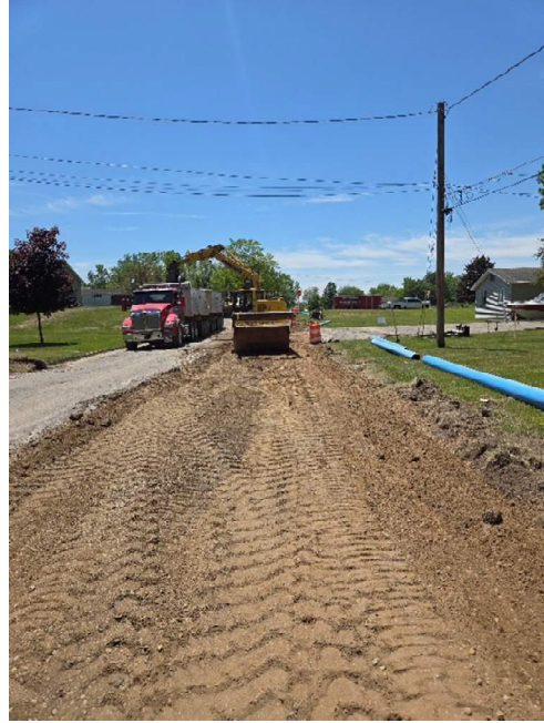
Photo 2: Phase #1 – Water Main installed on Essex and on S. Mill Street.
