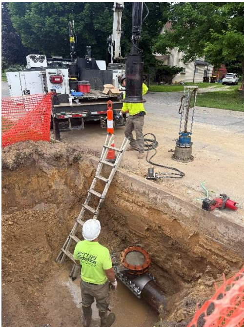
Photo 3: Phase #2 – Line-stops utilized to finalize water main tie-ins on Corinth Street.
