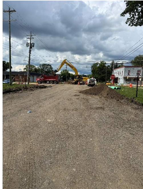
Photo 2: MDOT LAP – Sanitary mainline installed on N. Main Street.
