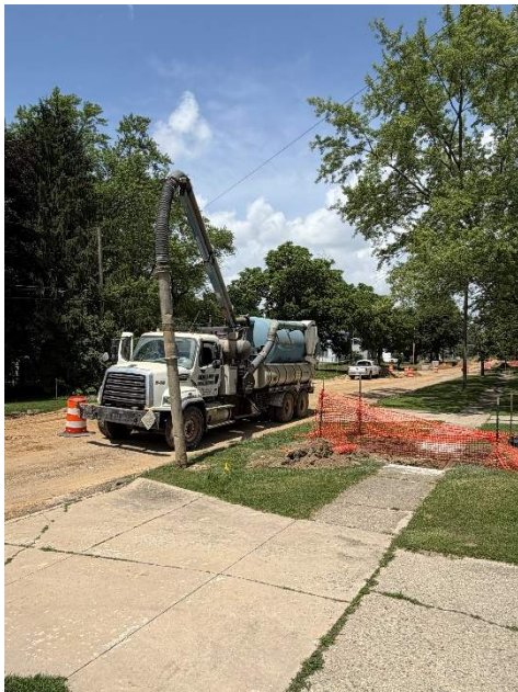
Photo 3: Phase #1 – Storm Sewer and water services placed on S. Mill and Essex.
