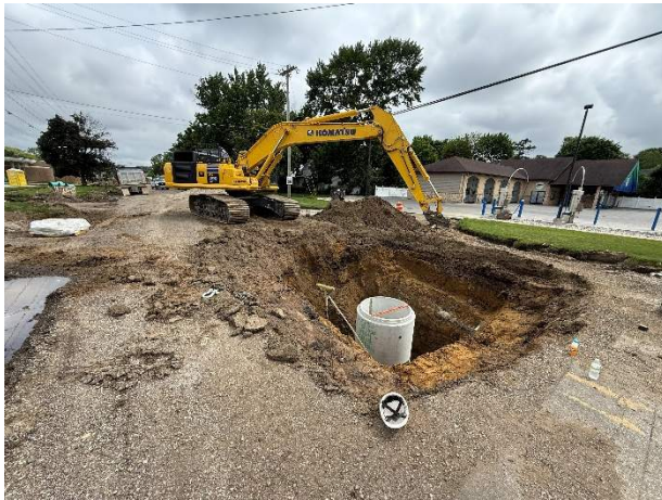
Photo 3: MDOT LAP – Temporary Sanitary manhole installed for bypass pumping.
