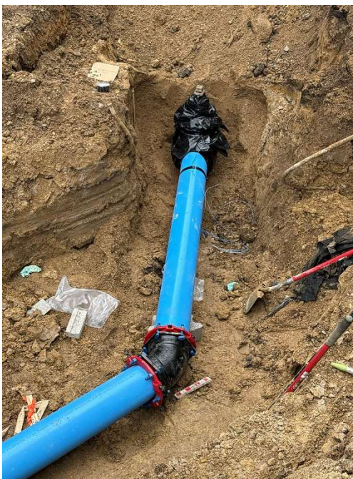
Photo 3: Phase #2 – Testing/chlorination, tie-in completed for watermain on Prospect.
