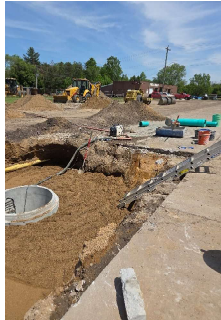
Photo 2: Phase #2 – Storm Sewer placed on Prospect Street.
