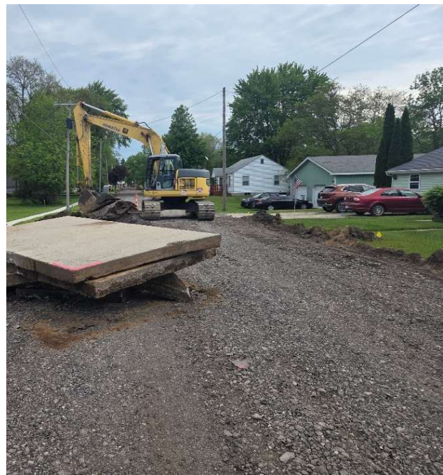
Photo 4: Phase #2 – Corinth Street pulverized and driveway removals started.
