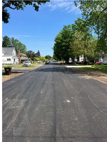
Photo 2: Phase #1 – Paving completed on N. Delaware and preliminary topsoil placed.
