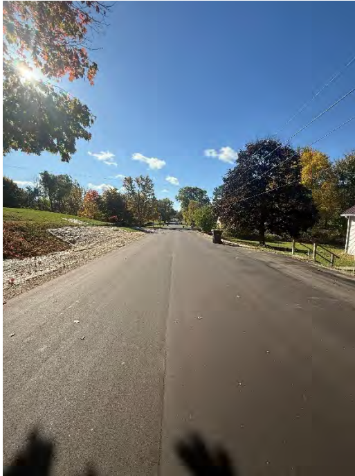
Photo 5: Contract #1 –Top course paving and restoration completed at Euclid.
