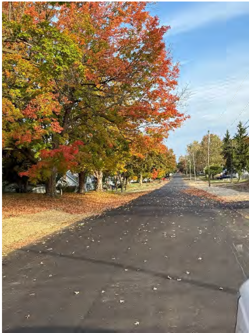
Photo 1: Contract #1 – Top Course paving and restoration completed at S. Franklin.
