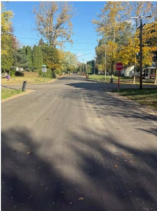
Photo 9: Contract #1 –Construction at S. Clinton street completed.
