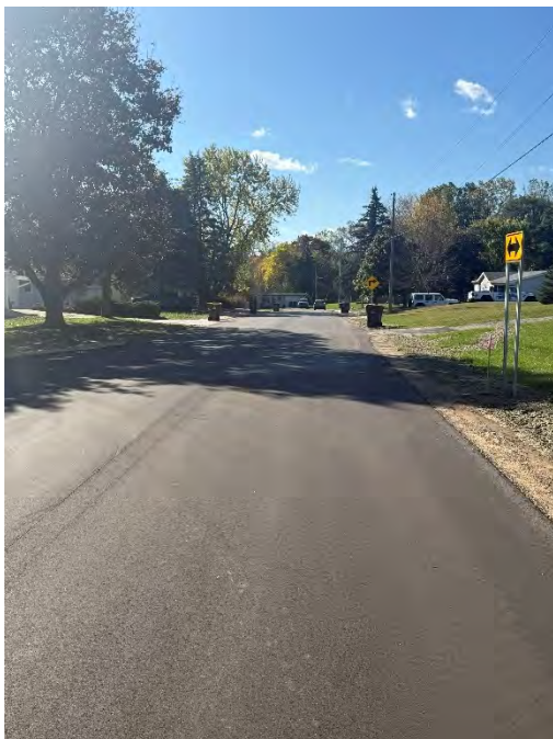
Photo 3: Contract #1 – Top course paving and restoration completed at East Street.
