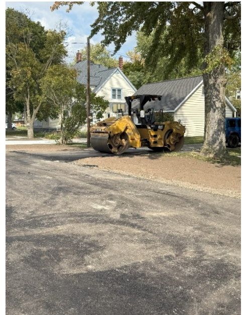
Photo 2: Contract #1 – Asphalt driveways placed on S. Franklin.
