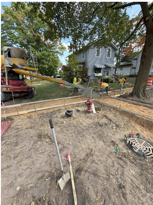
Photo 3: Contract #1 – Concrete Sidewalk ramps placed at Tyrell/Franklin.
