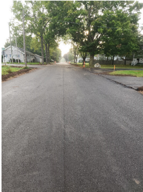
Photo 1: Contract #1 – Base paving completed at E. State Street.
