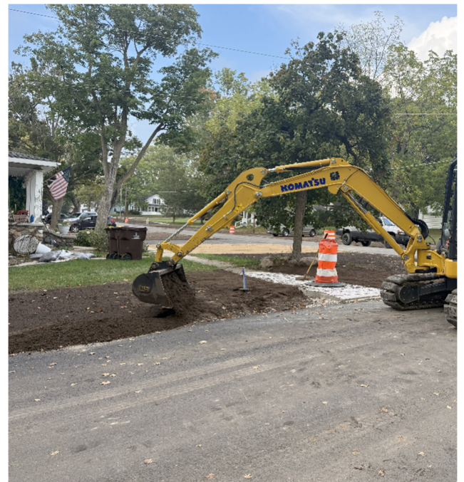
Photo 4: Contract #1 – Topsoil placed at S. Franklin Street.
