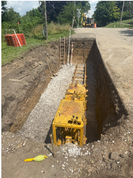
Photo 1: Contract #1 – Water Main Jack and Bore completed under Euclid.
