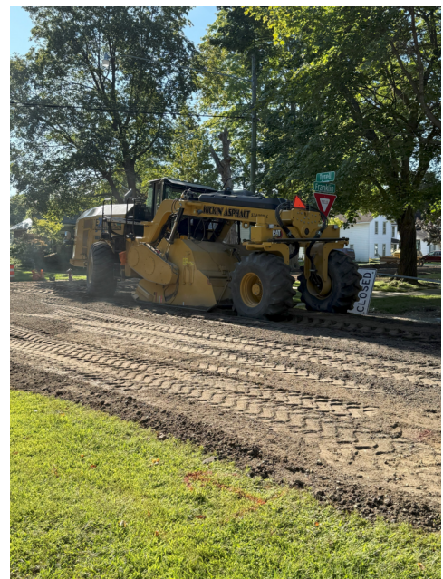
Photo 4: Contract #1 – S. Franklin overlayed with aggregate and road crushed.
