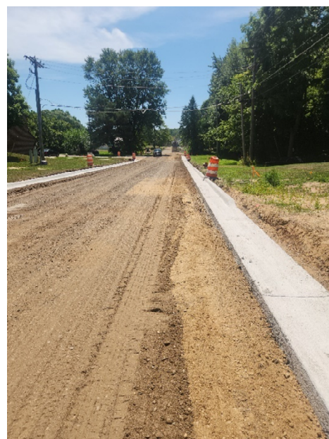
Photo 4: Contract #1 – Curb and Gutter placed on Euclid at the Oakridge apartments.
