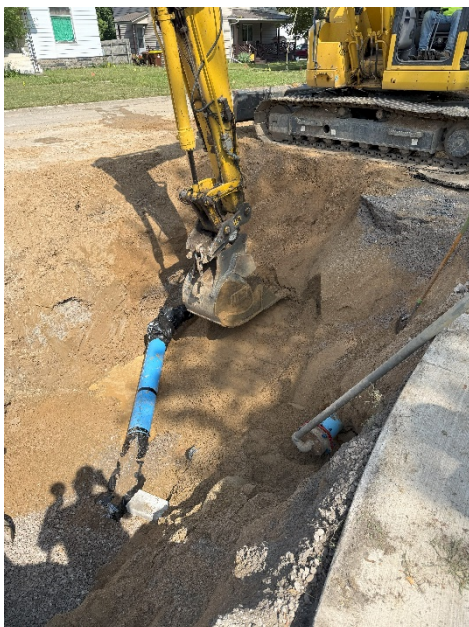
Photo 3: Contract #1 – Watermain tie-in completed at N. Franklin/Washington.
