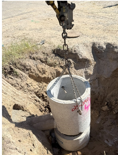
Photo 2: Contract #1 – Drainage Structures placed at Clinton adjacent to the tracks.
