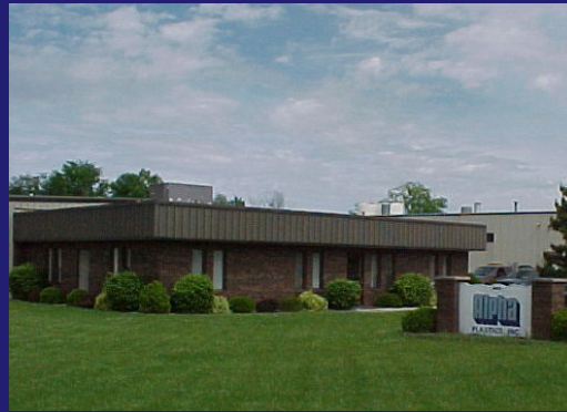
Alpha Plastics, Inc. (pictured above) was one of the first companies to build their business in the Woodside Industrial Centre in the Spring of 1986 and has expanded four times since then.
